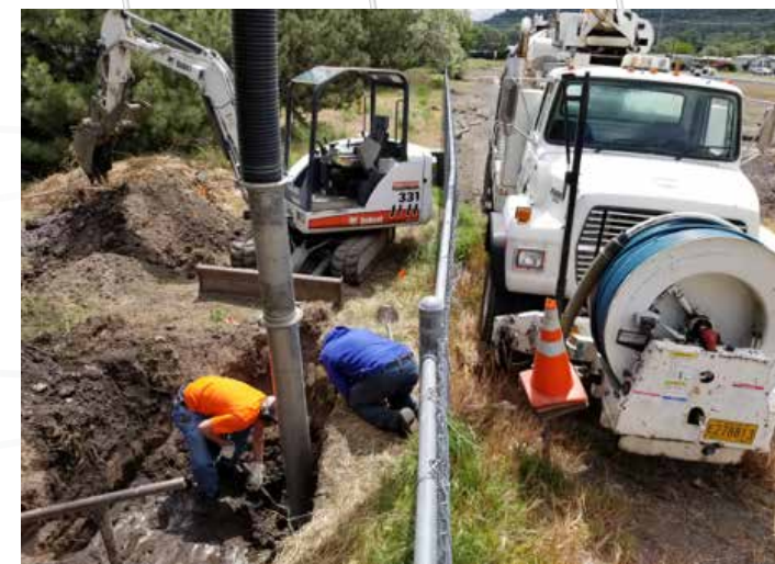
« New equipment helps in the fight against contamination as well. In the photo, the crew is using the new vacuum truck purchased this year. The vacuum truck assists in keeping the ditch clear of water while the workers make repairs.
